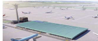
Located on the West of Passenger Terminal 2 control tower
