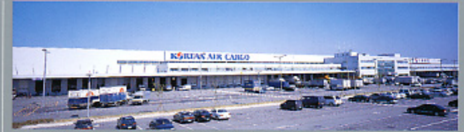
Incheon International Airport near Seoul
